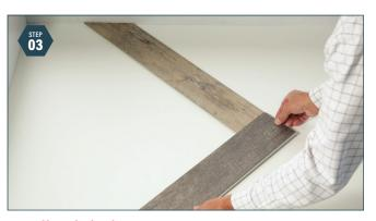
**Install 2nd plank** Take a second plank (B) and drop it with the long side engaging against the first plank (A) on the short side.
