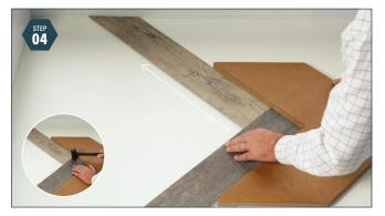
Align and lock Use the T-square to align the two planks perfectly. Then, tap gently with the soft rubber mallet to lock the planks.
