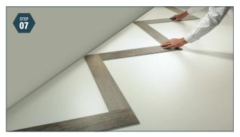
**Align row against wall** After finishing the first row of assembled planks, push it gently all the way against the wall.
