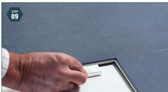
**Using disassembling wedge**
