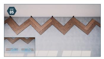
Prepare the end panels on each side. Use a 45° square to cut the panel and remove the excess.
